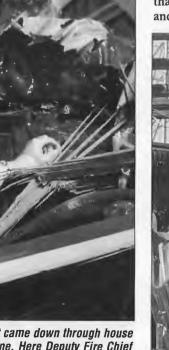
Only round to cause more than souvenir damage was one that came down through house on No. 17 and cracked pump gearbox, but did not put it off-line. Here Deputy Fire Chief Albert Brotherton inspects holes from shell fragments. (right) Capt. Hagen shows reporters tin roofing damaged by shell fragments. In background is splintered catwalk. After war, "Timbers" restaurant was built, featuring such damaged lumber as historical décor.
